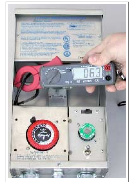
Photo 2 Testing Amperage
