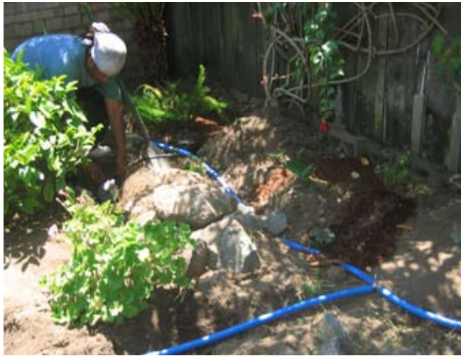
1-inch Blu-lock HDPE tubing laid out in trenches. All tubing was buried after system was finished. Photo: Laura Allen.
