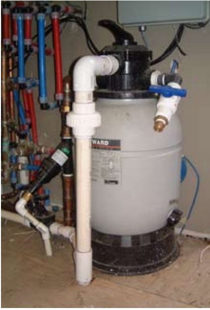
Graywater sand filter at the Sunset San Francisco Idea House. Photo: WaterSprout.
